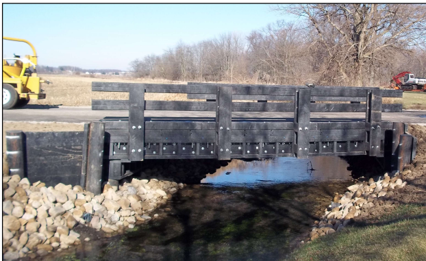
Bridge 174-0.56 over the Onion Ditch
